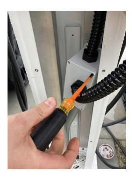
5. Use a multimeter to ensure that wires supplying power to the pedestal indicates a zero voltage, as there may be more than one circuit in the junction box.
