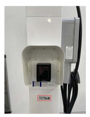
2. Peel off the backing paper from the CTEP label and stick the CTEP label below the pedestal label.
